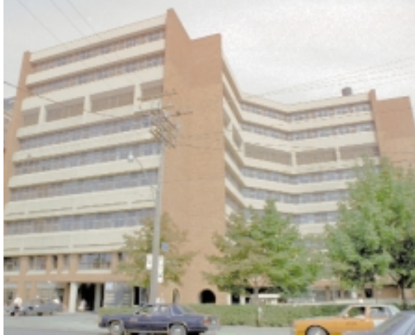
Toronto Western Hospital
